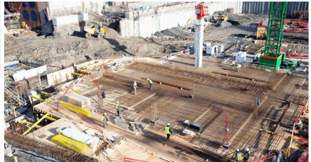
A view of the construction site of The National Children's Hospital. Photograph: Tom Honan/The Irish Times.
